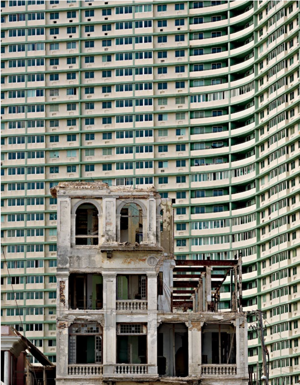
Partially demolished building with Edificio FOCSA in the background, Vedado neighborhood; Havana, Cuba; 2009; photograph © Richard Sexton
