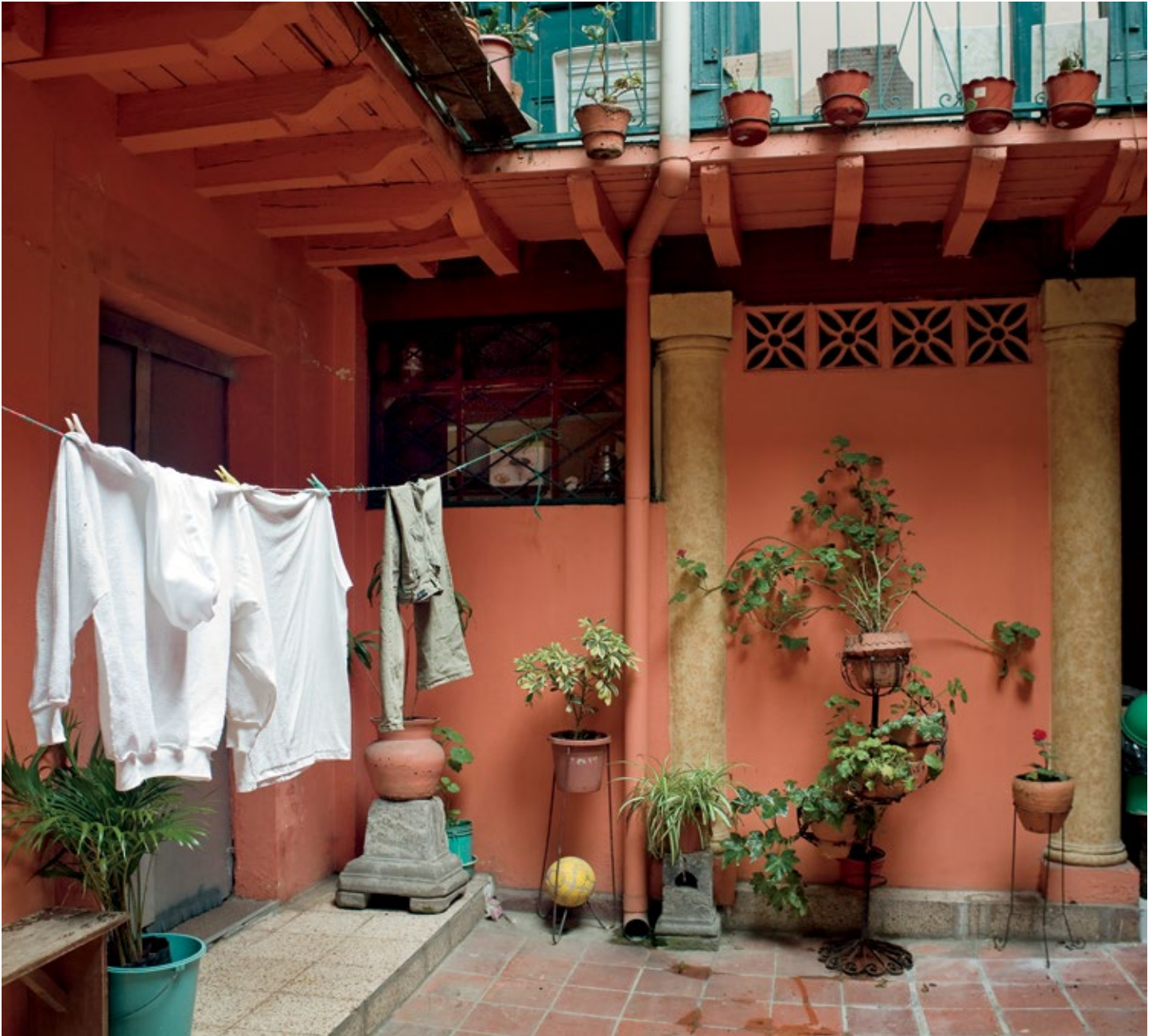
Courtyard, detail; Quito, Ecuador; 2008; photograph © Richard Sexton
